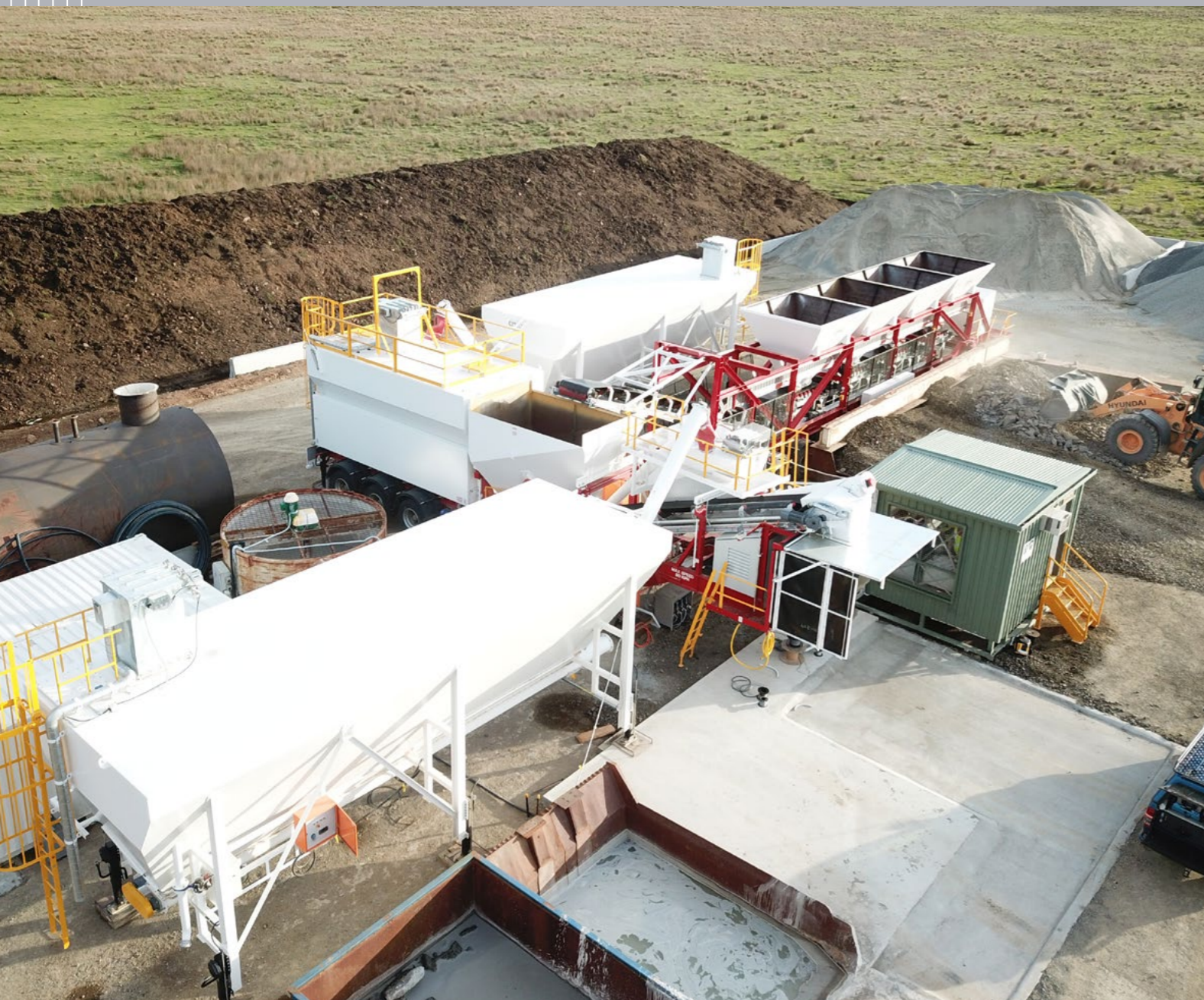
4-bin trailer, Portabatch and mobile silo set up
