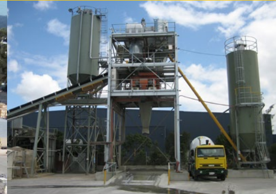
Twin shaft wet mix plant 100m 3 /hr
