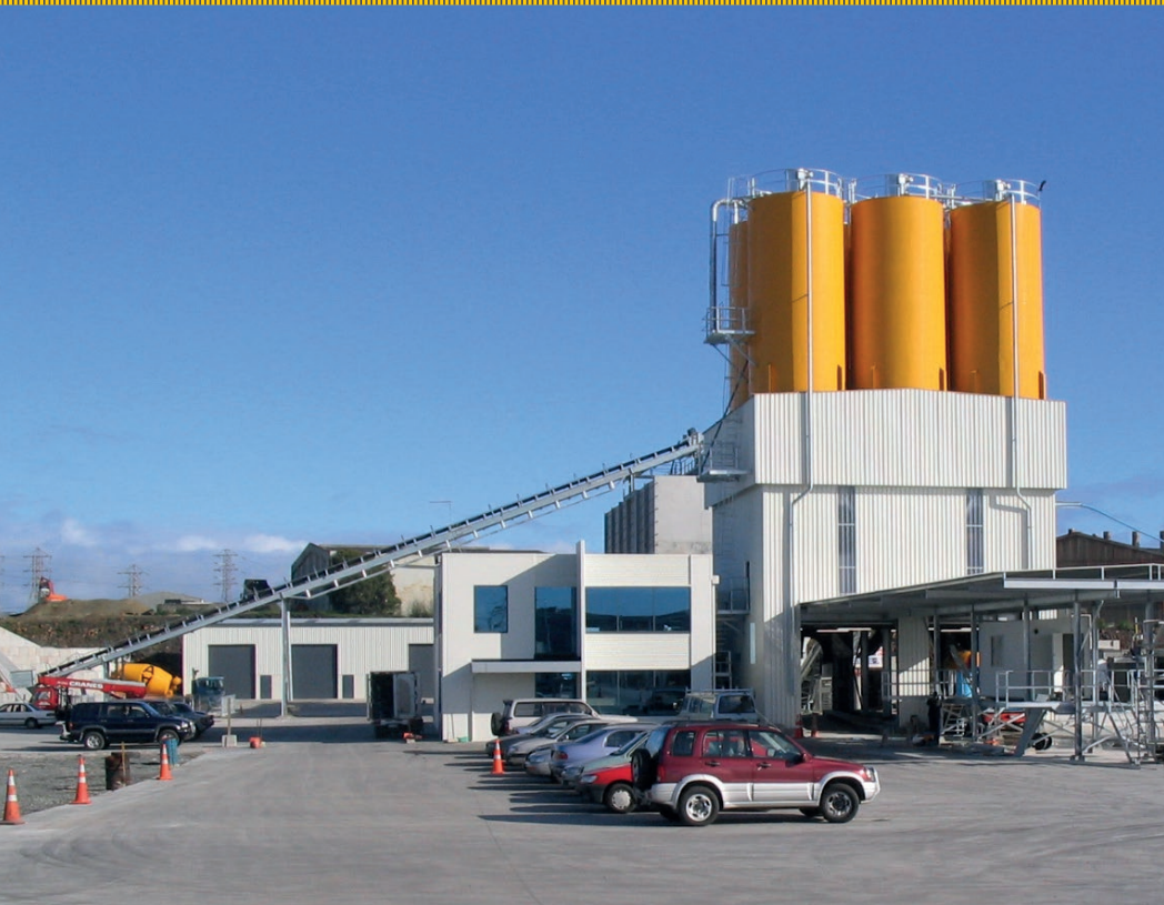
Dual alley plant 3,000T aggregate storage, 720T cement powder storage 360m 3 /hr
