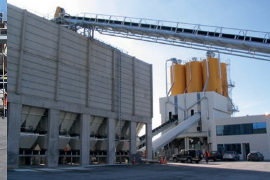
Dual alley plant 3,000T aggregate storage, 720T cement powder storage 360m 3 /hr
