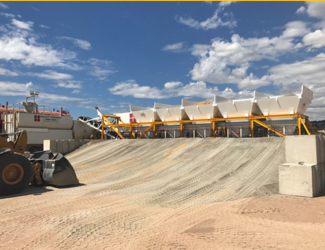
5 Bin aggregate trailer with belt weighers
